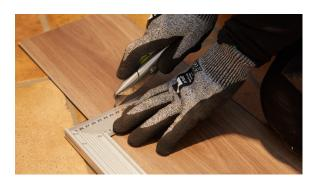
In places where it is too difficult to install the LayRed® panels with the tapping block (e.g. against the wall), you can tap them together using the pullbar and a hammer.
