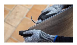
Put the panel with cut-off sides against the walls. Use the spacers to fill out the contour of the wall so that the panels do not move, are straight and are 100% installed and locked together correctly.
